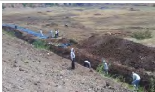
Percolation tank prepared at Hiwara, Jalna
